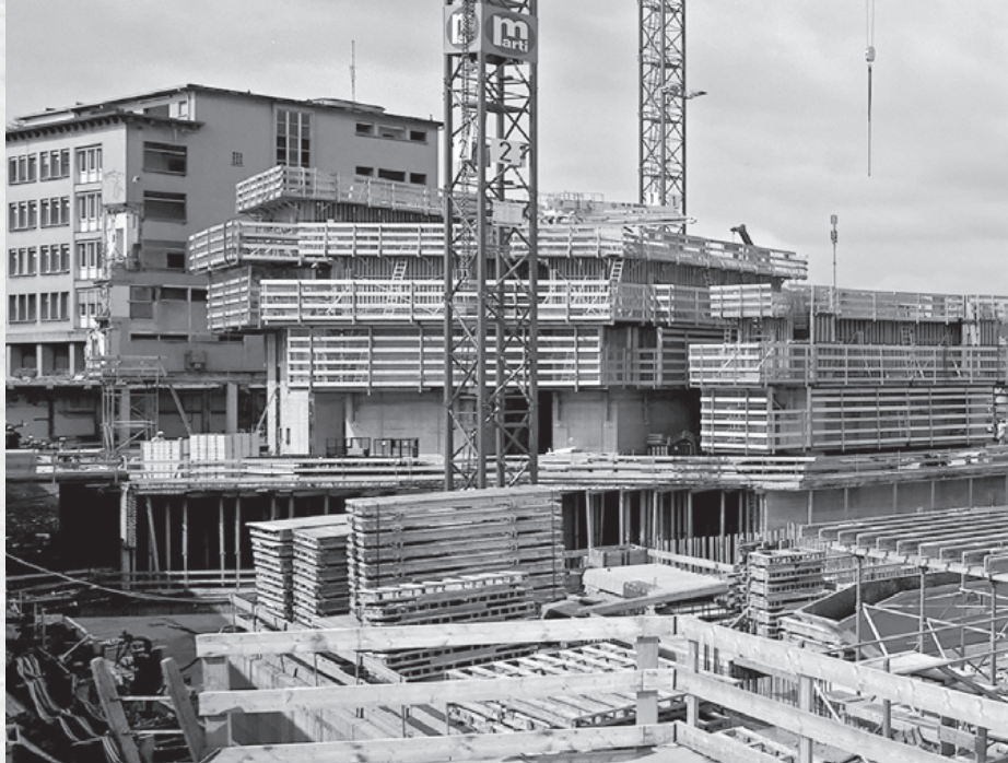
2008 Bau Prime Tower 34
