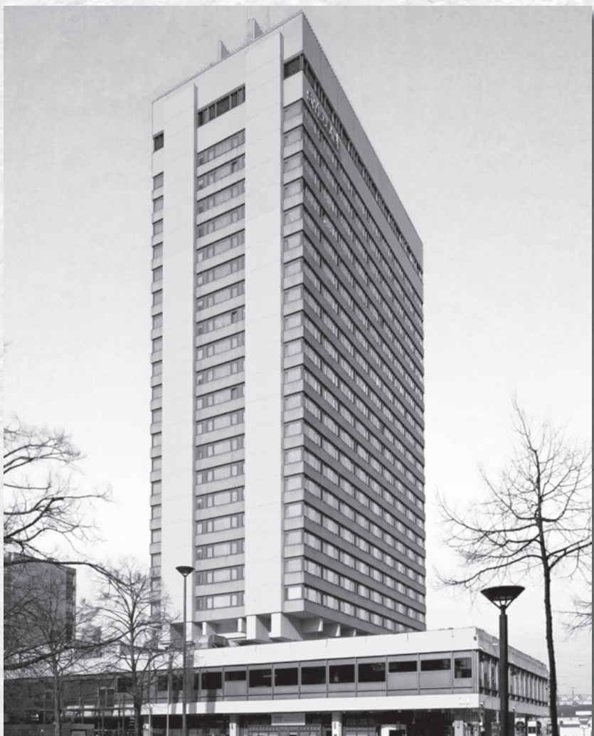
1972 Bau Hotel Swissôtel International 28
